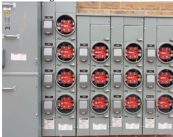
11.3 200 Amp, UD Multi-Gang Socket, Above 6 Positions
