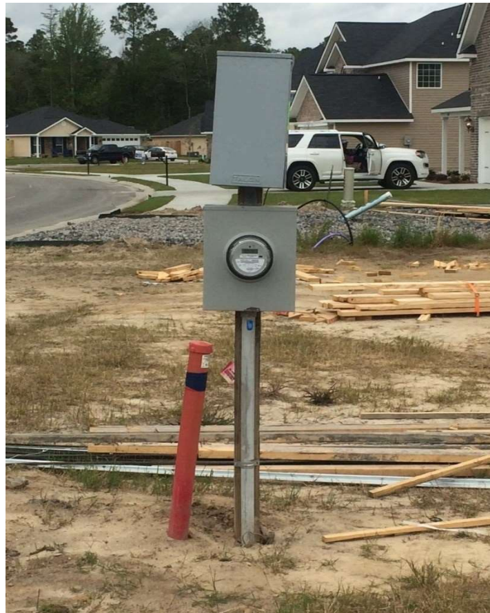
4.2 UD Temporary Service Installation
