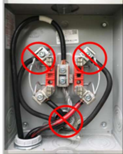
Improper routing of wires in the meter compartment, which does not allow proper clearance around the socket
