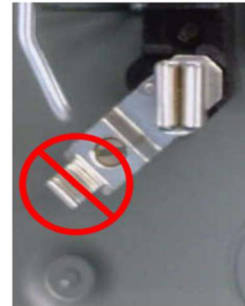
Socket lugs with factory “bypass horns”
