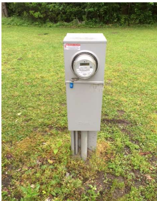
9.0 200 Amp, Customer Owned, UD Single-Phase Residential Socket
