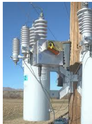
Hydraulic recloser – single phase application
