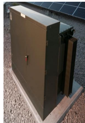
Three Phase Padmount Transformer
